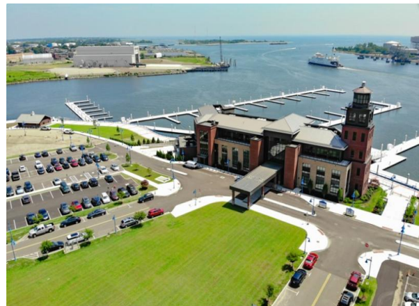
Steelpoint Harbor Development
