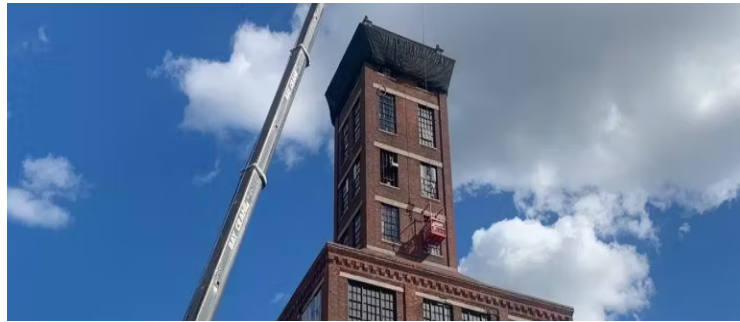
Demolition: Remington Facilities
