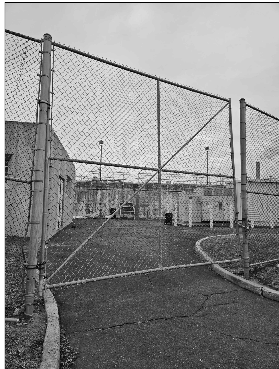
IMAGE 4: REPLACE SWING GATE TO REDUCE GAP TO PAVEMENT TO 6" MAXIMUM
