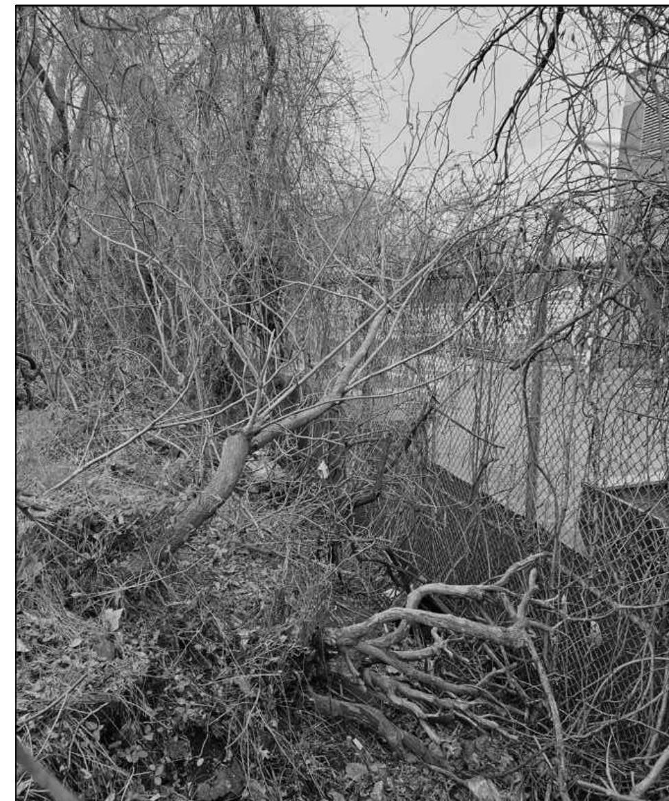
IMAGE 5: VINES AND VEGETATION TO BE MANAGED ONLY TO REMOVE EXISTING FENCE (PHOTO FROM ADJACENT PROPERTY) ALONG FENCE AT PROPERTY LINE, SEE SHEET C-04
