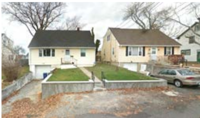
Figure 3.100-G. Basement Garage on House B Building
