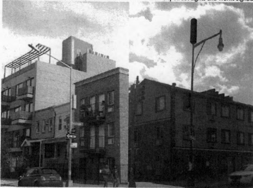
New York City Approved Pole Top and Cabinet Installations on City Street Lights and Traffic Signals
