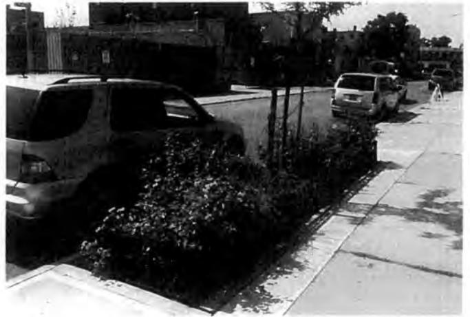
4) A typical bio-swale for Bridgeport
