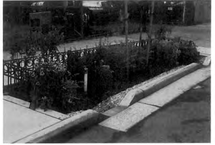
2) Here is shown the curb profile that lets gutter water detour into a planter where it can infiltrate or deposit pollutants and suspended solids (clay, sand, gravel, etc.).
