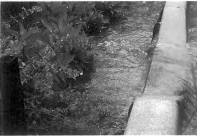
3) This image shows a rain garden or bio-swale emptying water that is filtered during a heavy downpour.
