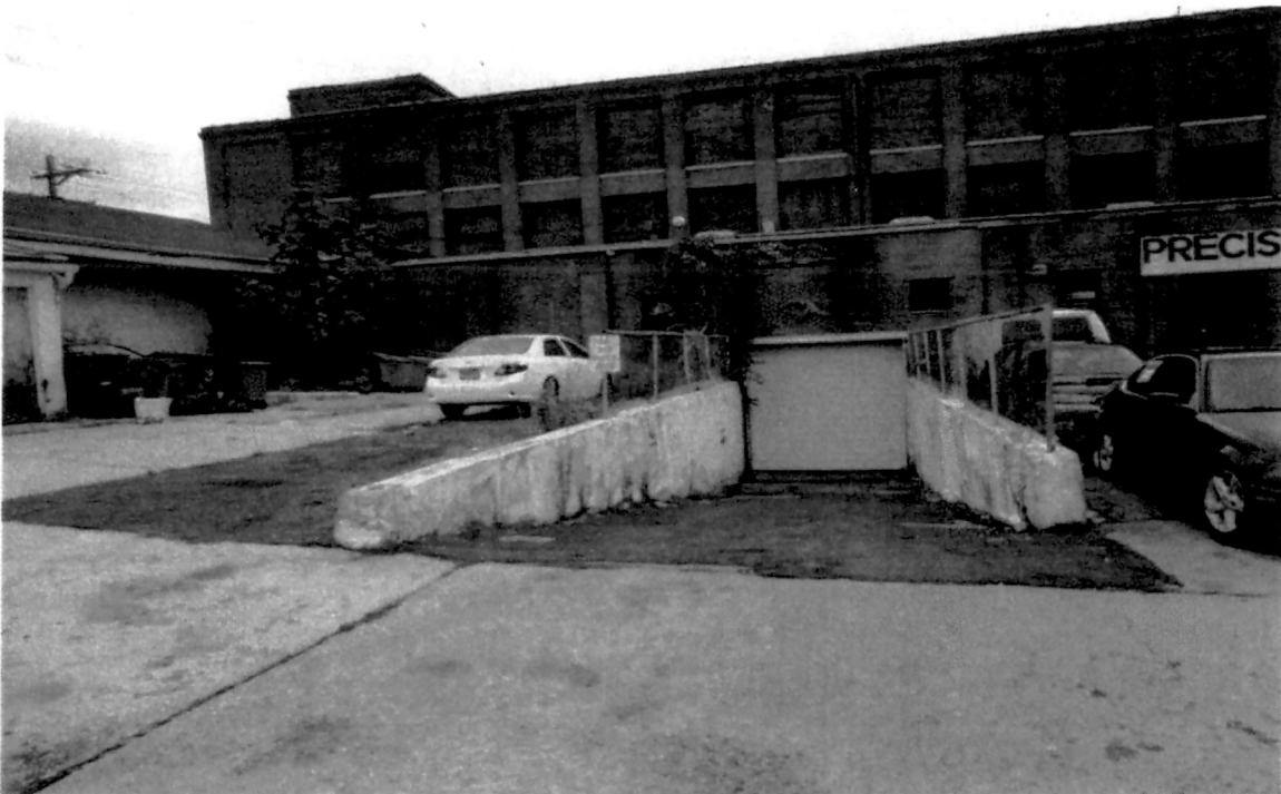
Ramp to basement auto storage
