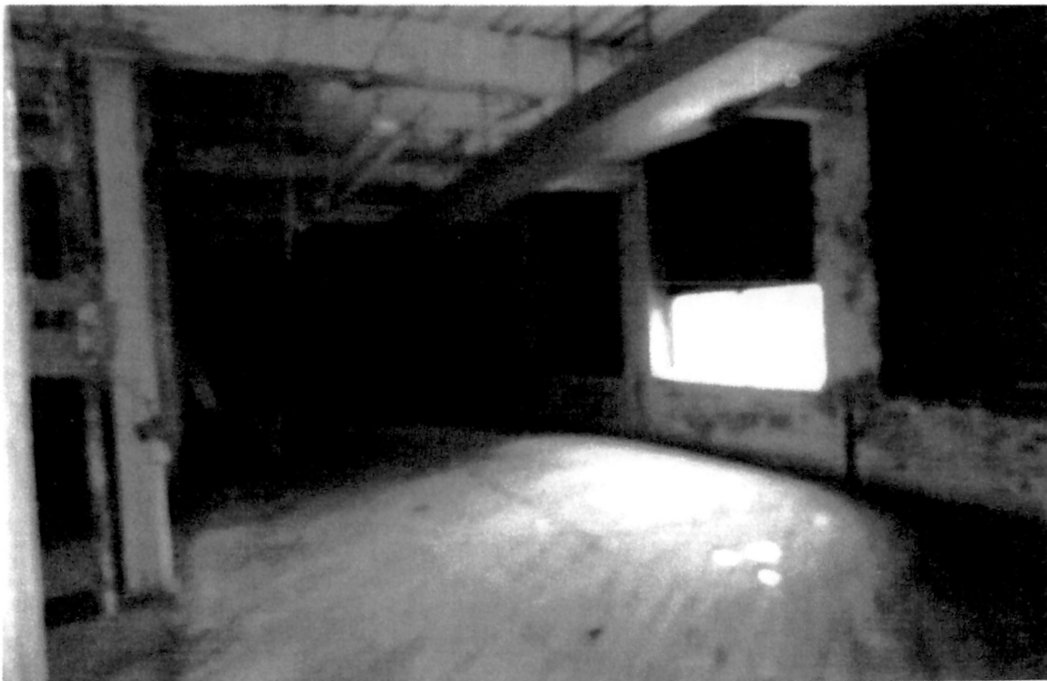
2 nd floor vacant
