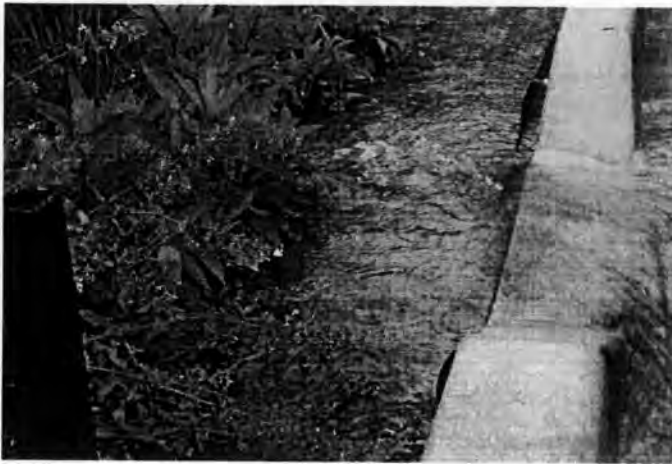
3) This image shows a rain garden or bio-swale emptying water that is filtered during a heavy downpour.
