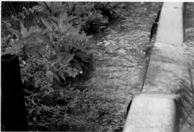
3) This image shows a rain garden or bio-swale emptying water that is filtered during a heavy downpour.
