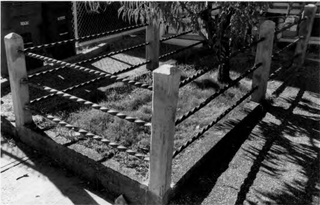
About ten years ago, the excavation for a house in BPT hit a buried foundation of a 100 year old structure that had this same twisted steel rebar for reinforcing. Perhaps at the same time it was installed for fences to protect the front yards of two large multifamily houses on Madison Avenue between Frank and George Streets. Today this small section is helping protect a peach tree.
