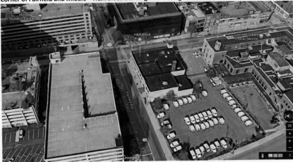
Corner of Fairfield and Middle – H&R Block Building Wall Facing Water Street
