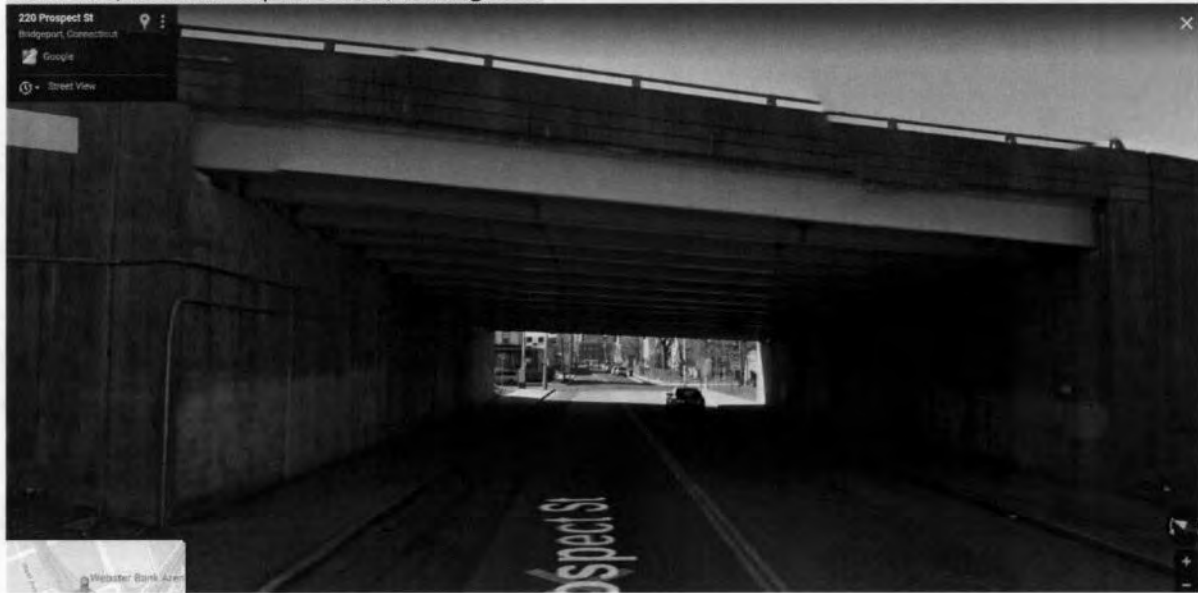
#8-A: Rt 8/25 and Prospect Street, looking west
