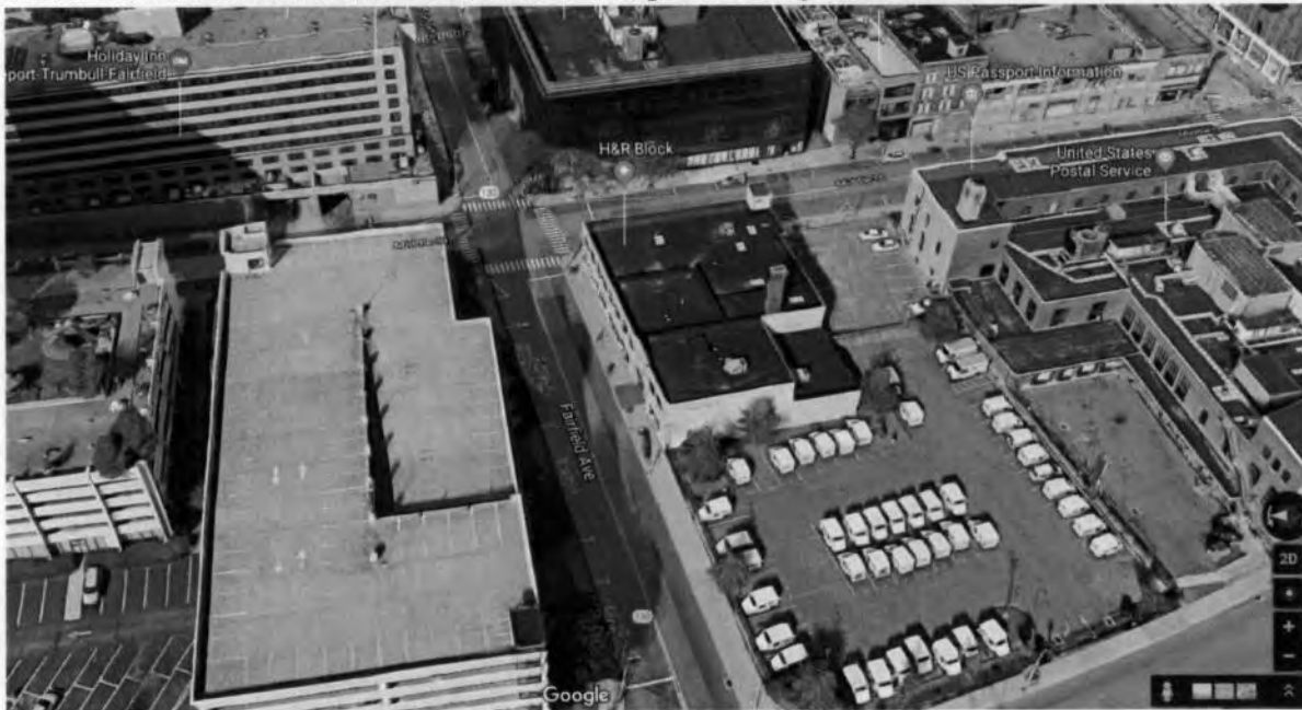
Corner of Fairfield and Middle – H&R Block Building Wall Facing Water Street
