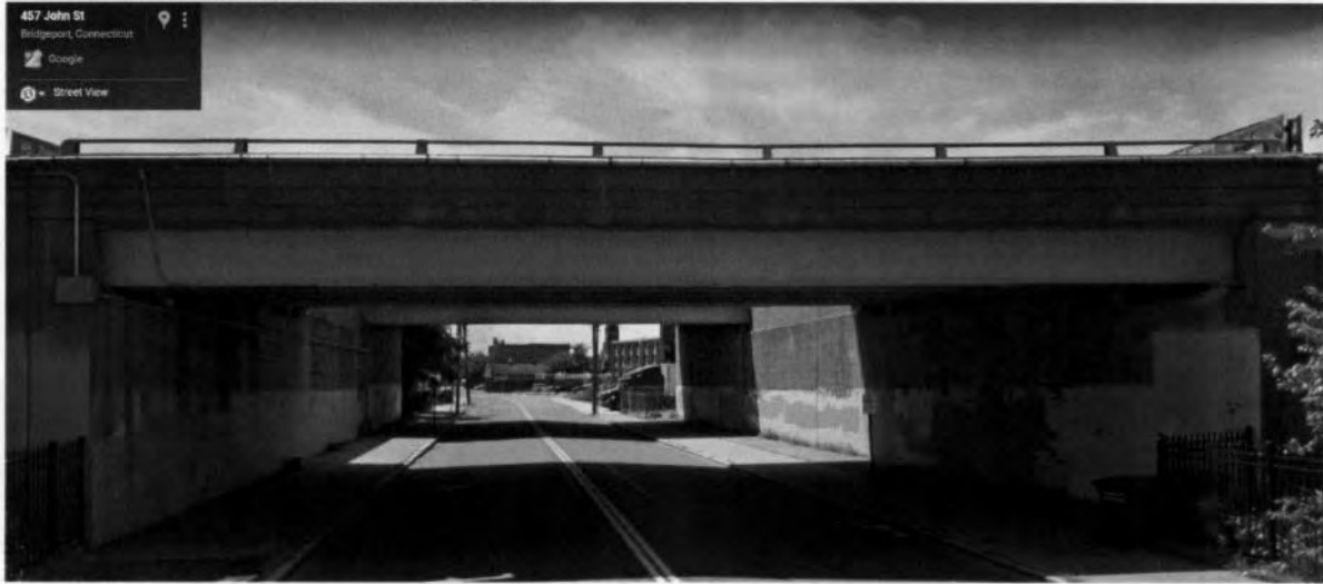
#8-C: Rt 8/25 and John Street, looking west
