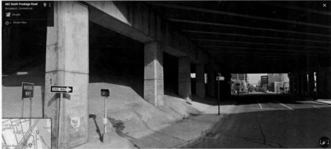
#95-G: I-95 and Main Street, looking north
