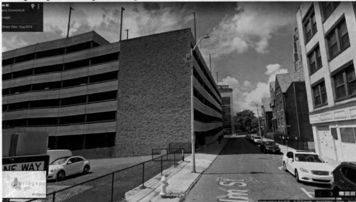
Parking Garage Wall Facing West Along Elm Street
