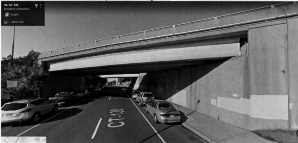
#8-D: Rt 8/25 and Fairfield Avenue (Rt 130), looking west
