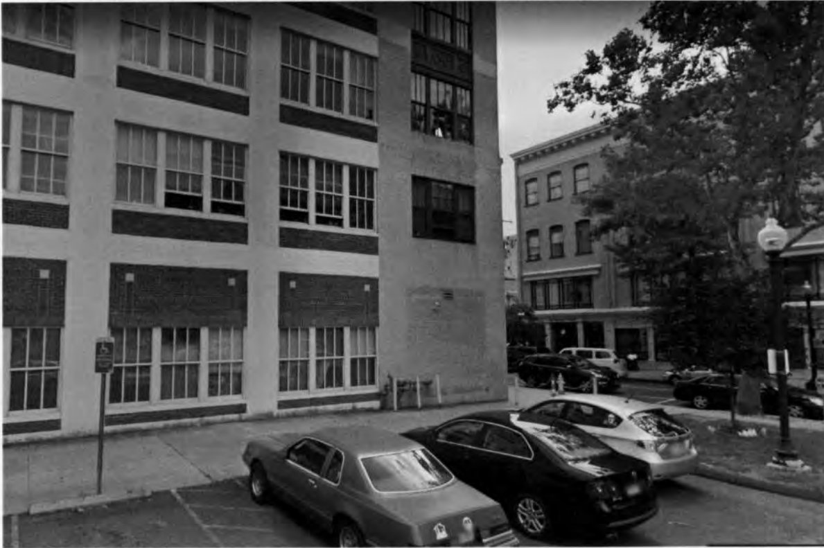
Reads Building on Broad – Framed Blank on Ground Floor Facing Cannon
