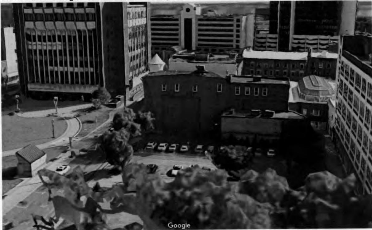
Old CT Post Building on Cannon Street – Facing Broad
