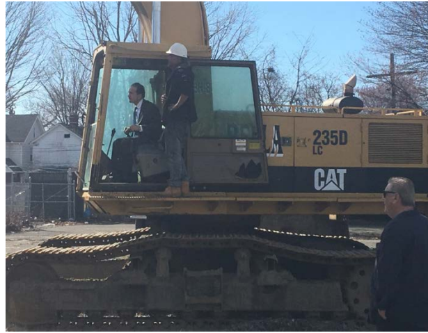
Mayor Joseph P. Ganim operating a tractor at worksite.
