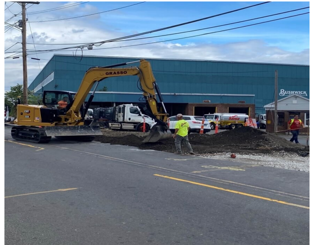
Construction of a shared use path on North Washington Ave.
