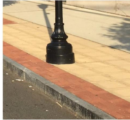
RED BRICK PAVING / COLORED SCORED CONCRETE
