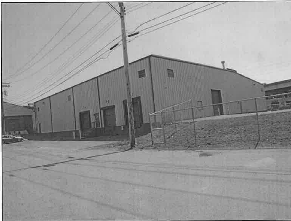
P4: Rear view of the studied building.
