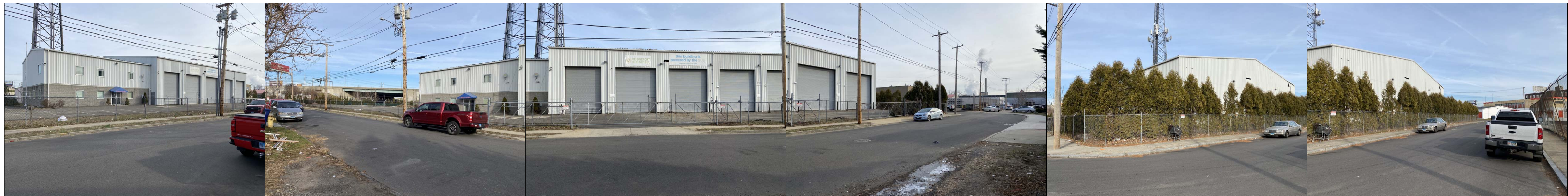
Andover Street & Bird Street Site Frontage - Fairfield Avenue to Bird Street
