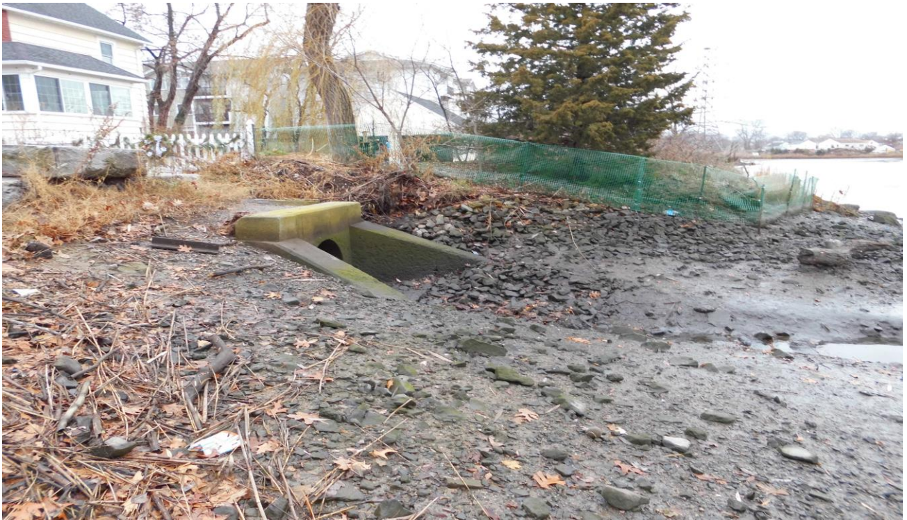
PHOTO 9: View of outfall at Davidson St, looking southwest.
