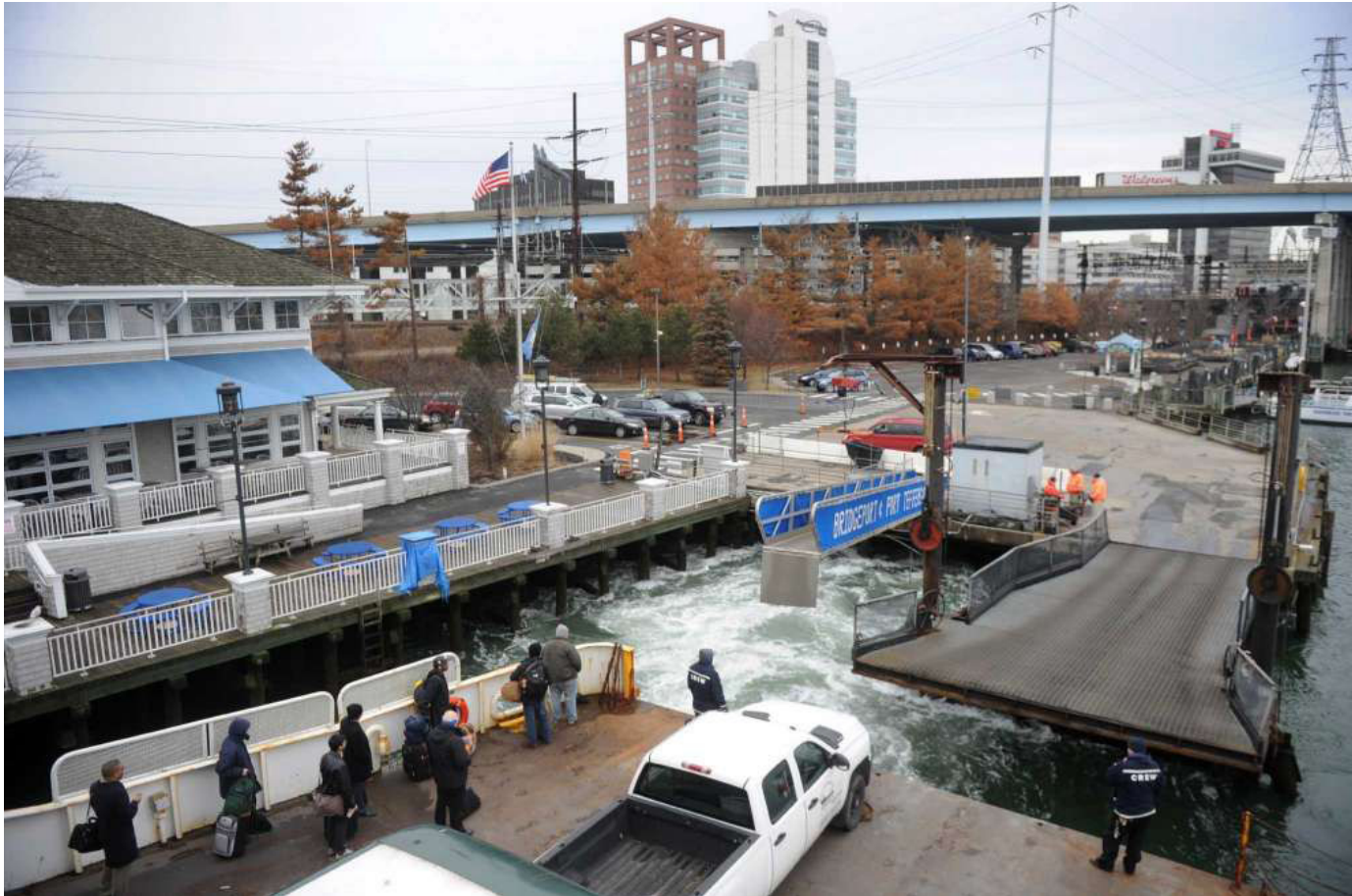
A short walk from Downtown Bridgeport, the train station, and the Harbor Yard sports complex with existing moorings, the current Port Jefferson Ferry Terminal site is a prime location for attracting visitors by boat. Image Source: Brian Pounds, CT Post
