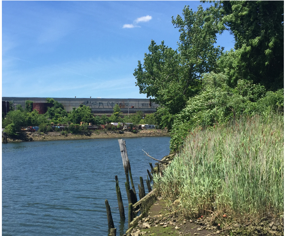
The recent construction of Bridgeport's Knowlton Park included a biofiltration swale with native grasses (above, on right) and a stretch of riparian buffer, both local examples of LID. Not only does the biofiltration swale create an attractive view for park visitors, it also protects the shoreline against erosion and the park itself from flooding.
