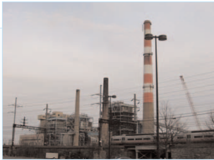
United Illuminating Power Plant (Bridgeport)
